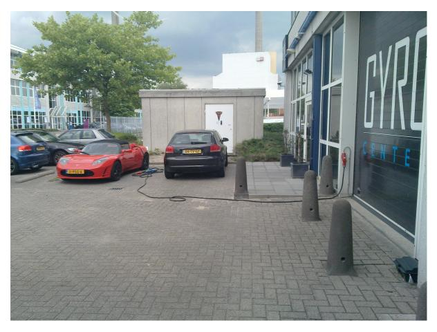
Various buildings have 3-phase connectors installed on the outside. In this case a 3x32A connector was mounted on the outside for general usage.
