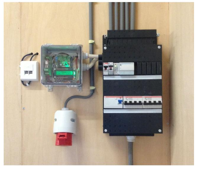
The red socket is the additional 16A 3-phase CEE socket I installed. It's not for the EVSE. I added a second 16A breaker on the top in case you noticed.
