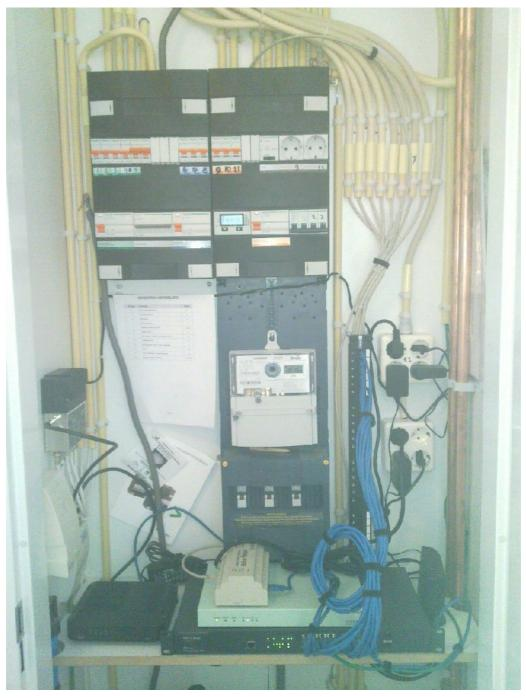
This is a total overview with my network wiring in there as well. On the bottom row of the panel you'll see the kWh meter and on the right the 32A breaker (in off position). The grey cable on the top is the one towards my shed.
