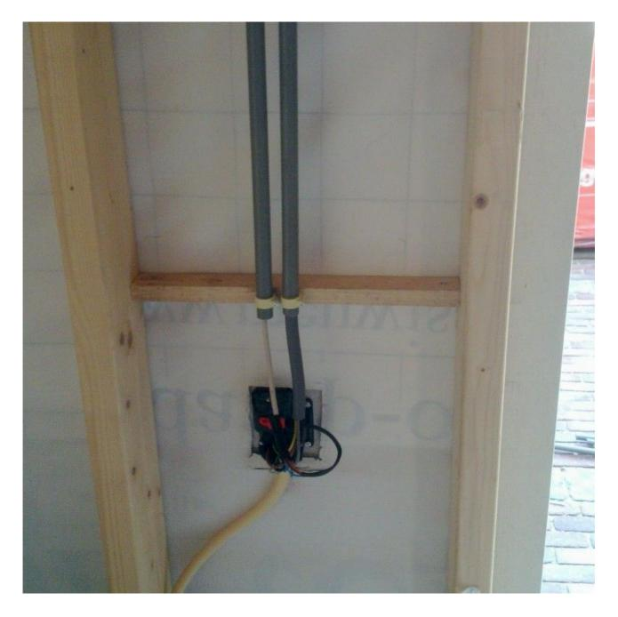
This is the back of the socket installed on the outer wall. You can see the interlocking actuator installed on top of the socket.
